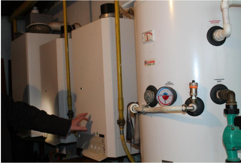
Photo 5 Gas boilers in the boiler house
