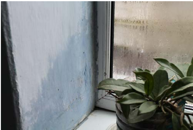
Photo 6 Consequences of the low ventilation level, first floor, classroom
