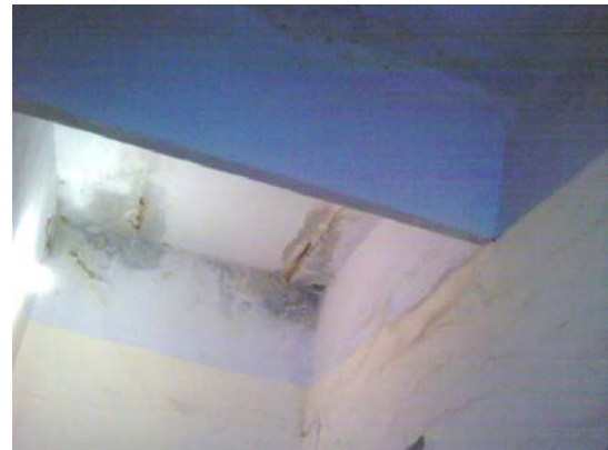
Photo 7 Signs of roof leaking in the corridor
