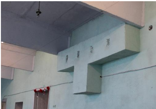
Photo 10 Vent holes in canteen
