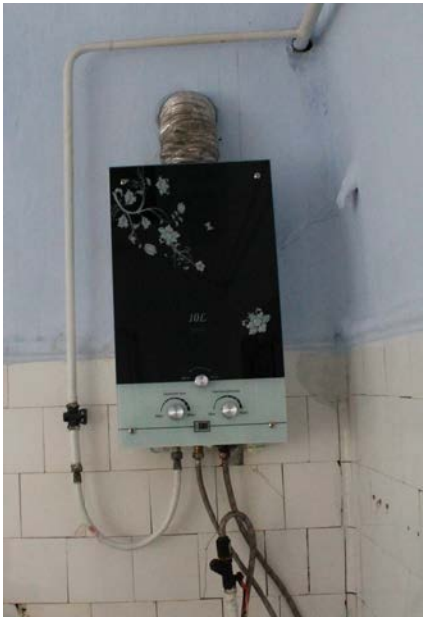
Photo 6 Gas water heater, in the kitchen.
