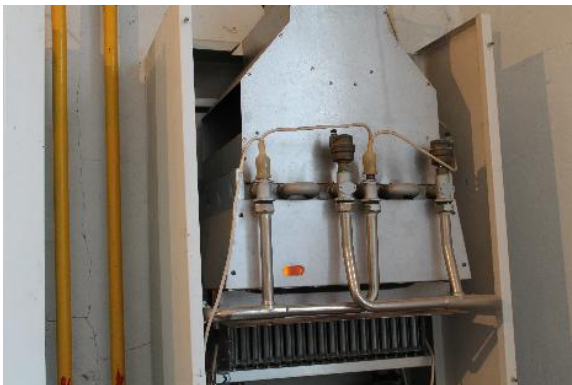
Photo 5 Gas boiler in the interior boiler house
