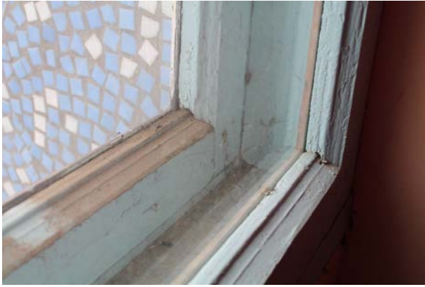
Photo 4 Double wooden framed window with one layer of glass
