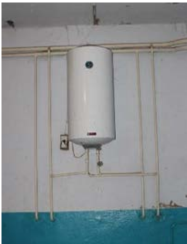
Photo 8 Electric boiler
