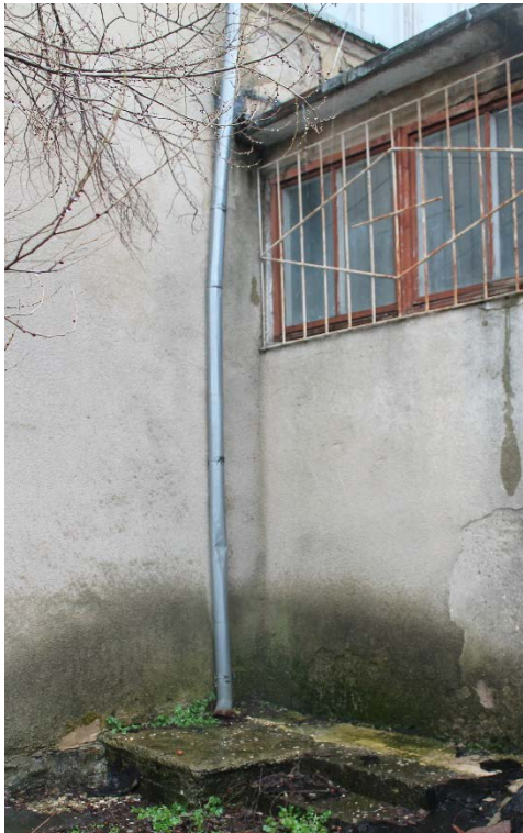
Photo 5 Rainwater drain, connection between block A and B
