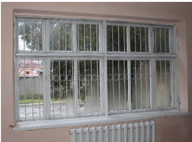
Photo 3 Wooden window, south façade
