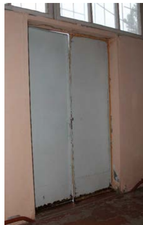
Photo 4 Auxiliary door, south façade
